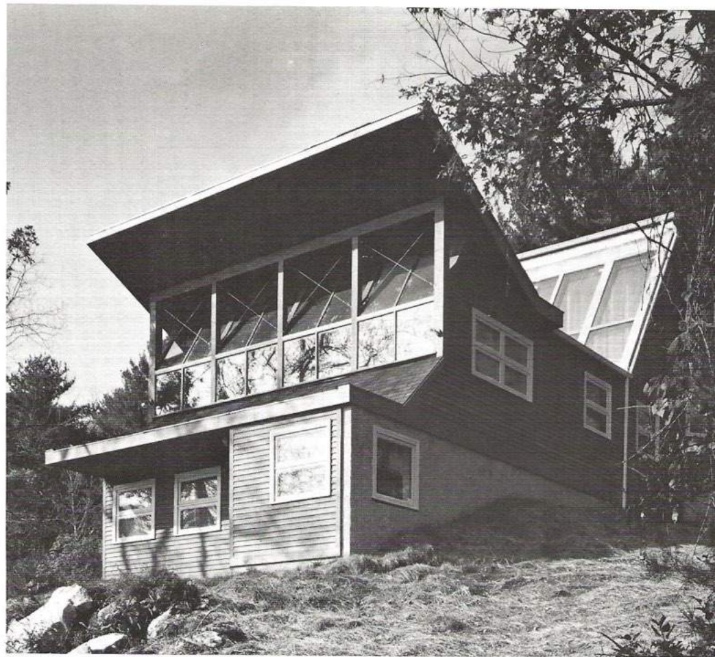
南東より見る View from southeast
