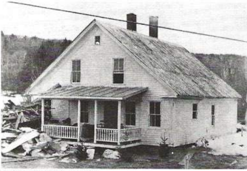
改造前 Before renovation
